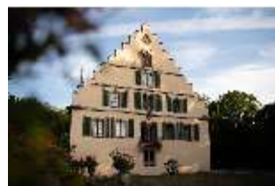
CoR.I, Nordfassade, DI025444, BSV-
