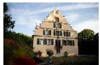
CoR.I, Nordfassade, DI025445, BSV-
